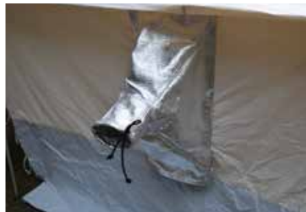
4) HEATER FLUE PIPE SLEEVE
